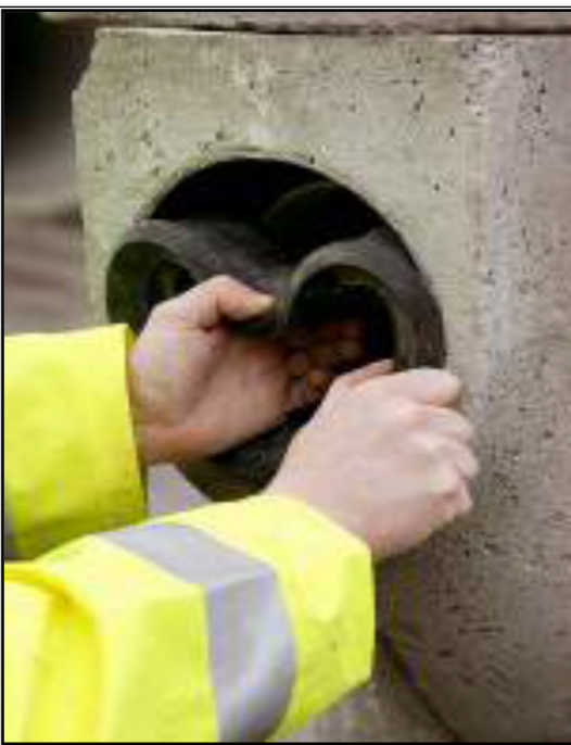
Rubber insert to be installed into gully traps for use with PVC pipes.
