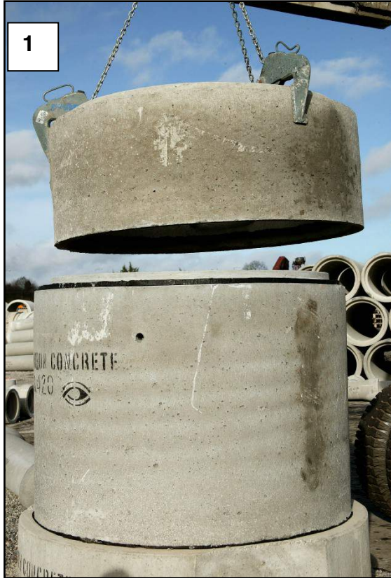
Positioning of 0.5M Chamber Ring
