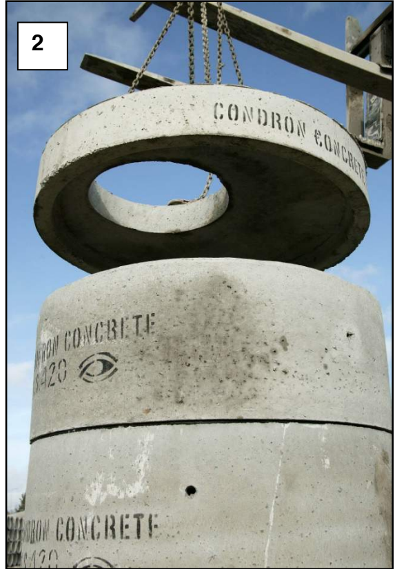
Positioning of Manhole Cover
